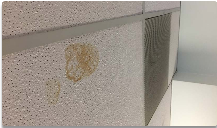
New Ceiling Tiles in offices
