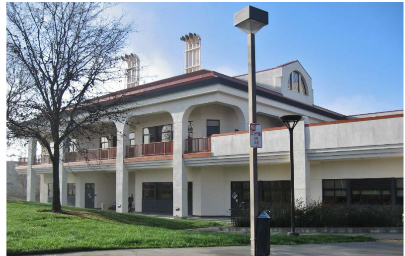
1997 Science & Tech classroom Building 1800 renovated in 2012
