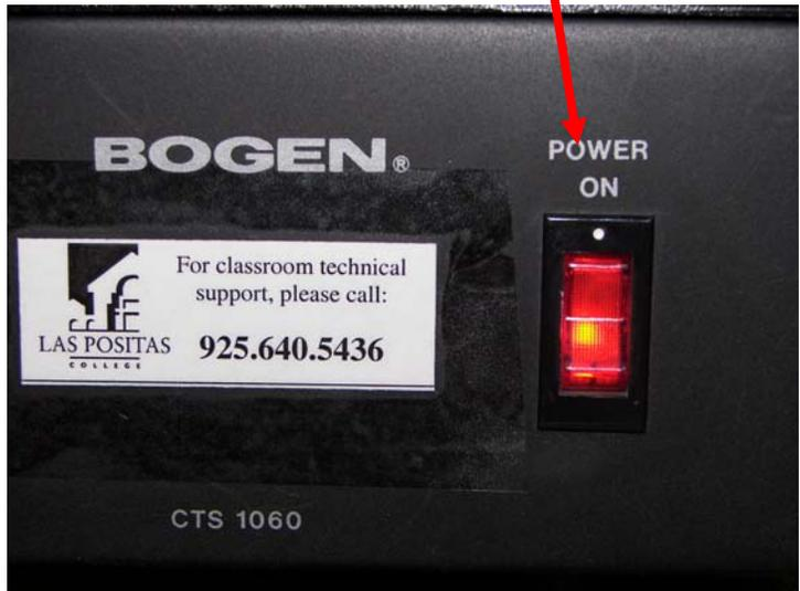
Turn on the audio amplifier unit located in the closet - the orange light will glow.
